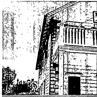
• Balconies with sawn wood railings
