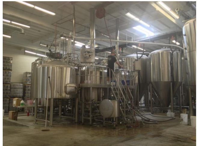
Production vessels at Coronado Brewing Co. in Bay Park
