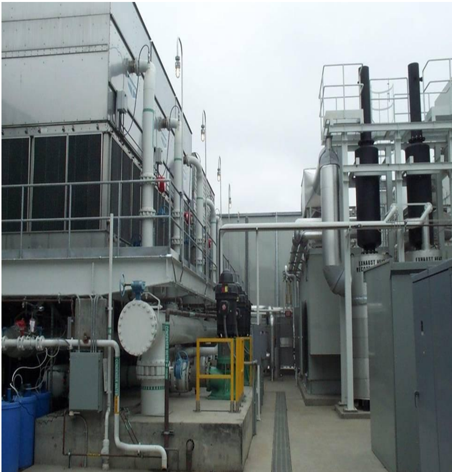
Johnson & Johnson's La Jolla R&D laboratory is cooled using reclaimed water
