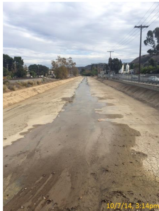
Photo 2. Sorrento Creek Reach 3 Post-Maintenance 10/7/14
