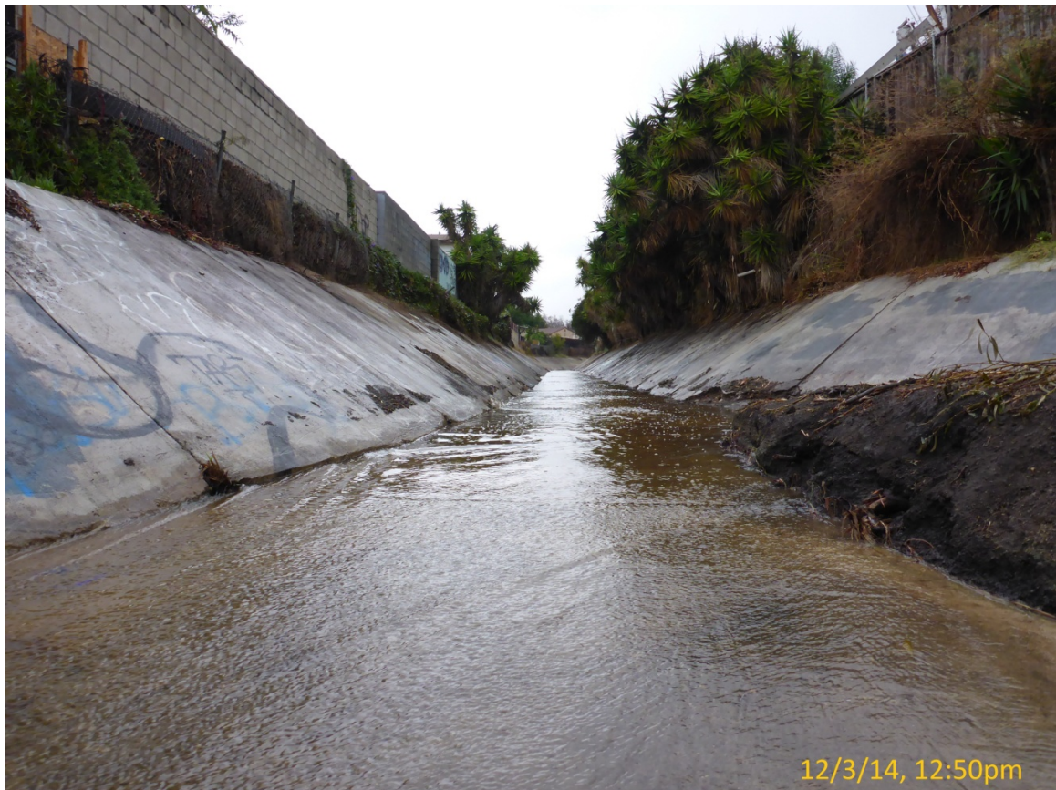
Photo 12: Smythe Channel Emergency Post-Maintenance 12/3/14
