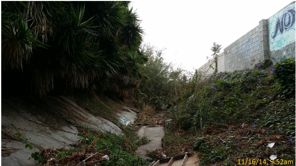
Photo 11: Smythe Channel Emergency Pre-Maintenance 11/16/14
