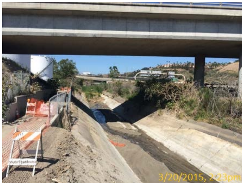
Photo 4. Murphy Canyon Creek Channel Post-Maintenance 3/20/15
