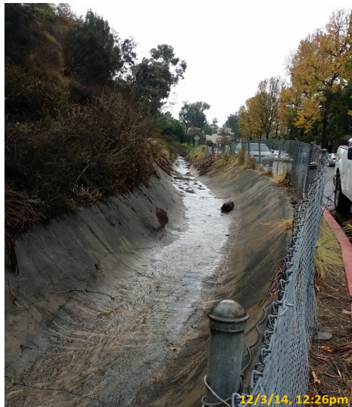
Photo 10: Reservoir Drive Channel Emergency Post-Maintenance 12/3/14
