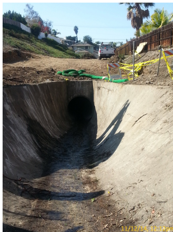
Photo 8: San Carlos Creek Channel Emergency Post-Maintenance 11/12/14
