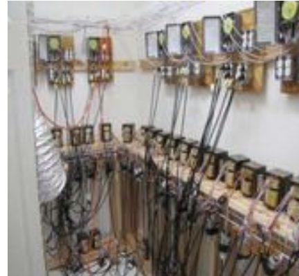
Residential Electrical Rewiring source: Chief Marc Vasquez.
