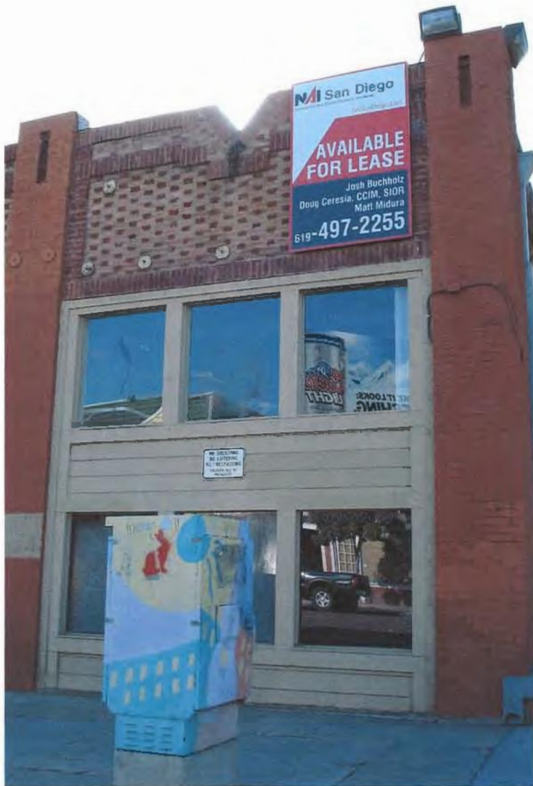
14. 741 F Street View to west of bay at north corner on east facade. New wood siding and windows. March 9, 2011
