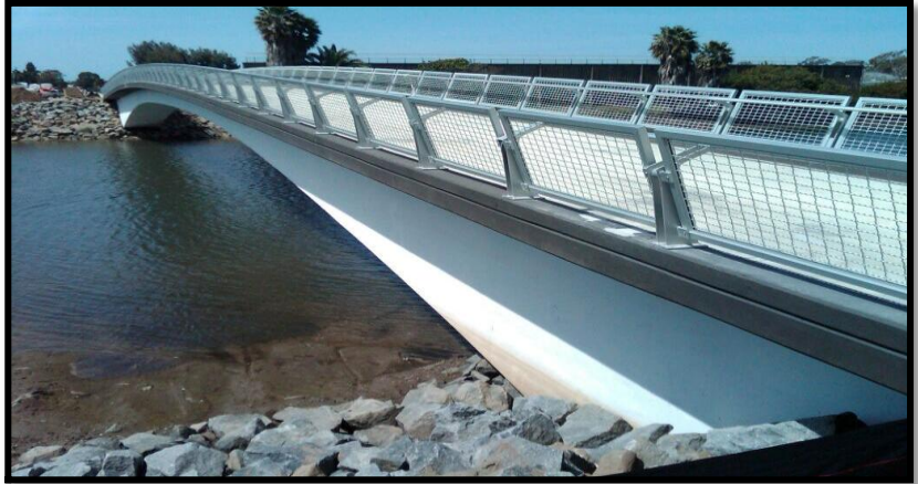
Rose Creek Bikeway and Pedestrian Bridge
