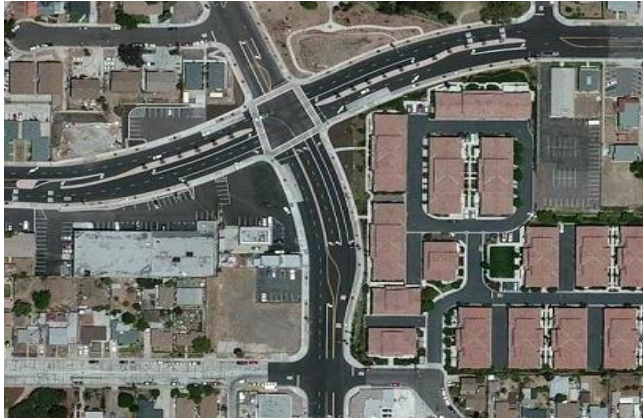
43rd Street & Logan Avenue Realignment
