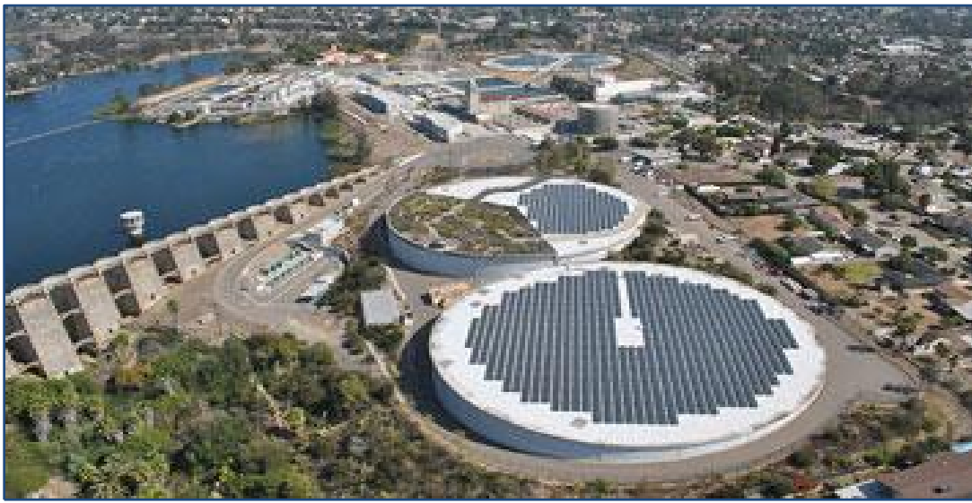
Alvarado Water Treatment Plant project
