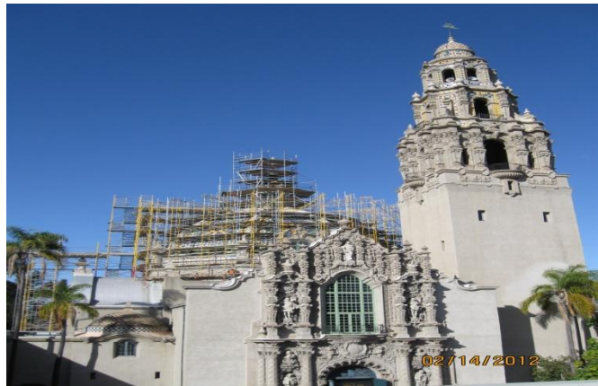
Museum of Man Dome Restoration & Repair
