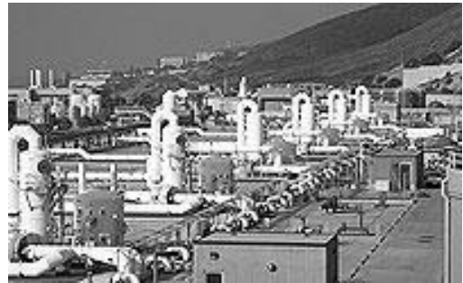
Photo 5: Point Loma Wastewater Treatment Plant
