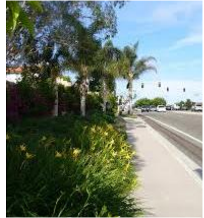
The photo shows a contiguous sidewalk. This design is strongly discouraged.
