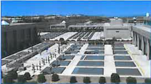
North City Water Reclamation Plant
