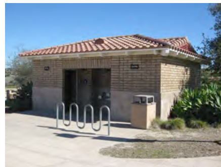
Facility 10370 – South Village Neighborhood Park Comfort Station
