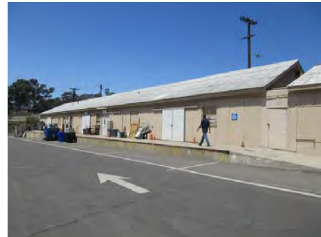
000033 - Fac. Maint., HVAC Shop
