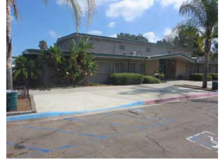
Facility 000480 - Recreation Center, Serra Mesa
