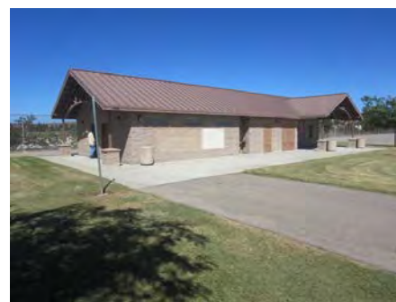
Facility 010420 - De Portola Mid Sch., Joint Use Area, Comfort Station
