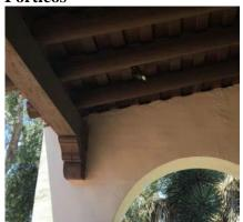
•Plastered adobe columns and wood beams and rafters
