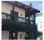
•Exposed rafters, purlins and rafter tails, clad with clay tiles
