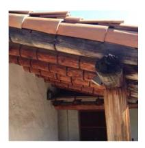
•Hand-hewn wood support posts, beams and rafters
