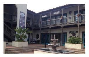
•Simple, heavy structure with wood support posts, beams and rafters, clad with clay tiles
