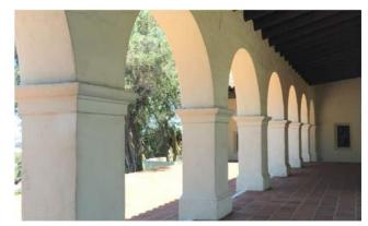
•The columns' uppermost molding serves as impost mold from which the arches spring
